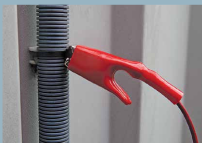
Small diameter cable tracing techniques
